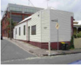
cremorne cubitt street cremorne cubitt street 167
