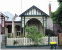
richmond malleson street richmond malleson street 8
