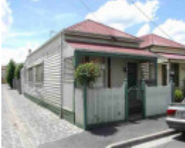
burnley kimber street burnley kimber street 1
