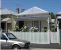
burnley kimber street burnley kimber street 6
