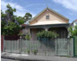
richmond miller street richmond miller street 13
