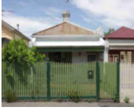
richmond miller street richmond miller street 15
