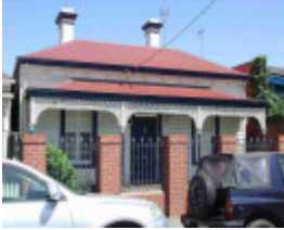
richmond miller street richmond miller street 16
