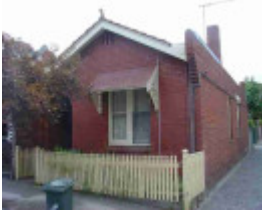
carlton north macpherson street carlton north macpherson street 70
