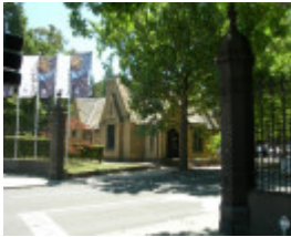
MAIN ENTRANCE GATES (GATE 6), PILLARS AND FENCE SOHE 2008
