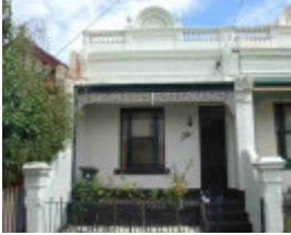
carlton north macpherson street carlton north macpherson street 135
