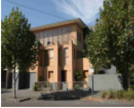
princes hill park street princes hill park street 544
