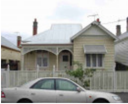
richmond malleson street richmond malleson street 24
