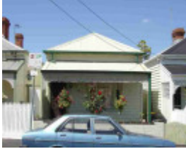
burnley kimber street burnley kimber street 14
