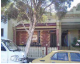
carlton north ogrady street carlton north ogrady street 52
