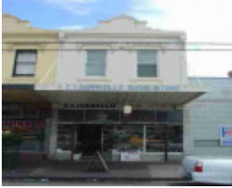
carlton north nicholson street carlton north nicholson street 725
