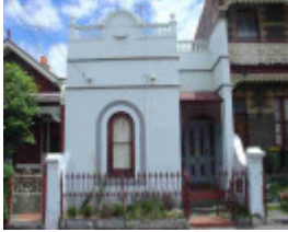
carlton north station street carlton north station street 217
