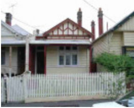
richmond malleson street richmond malleson street 16
