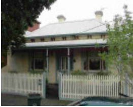
richmond charles street richmond charles street 55
