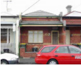
richmond yorkshire street richmond yorkshire street 31
