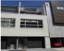
richmond wangaratta street richmond wangaratta street 18
