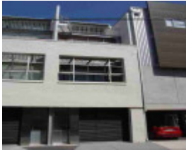
richmond wangaratta street richmond wangaratta street 18
