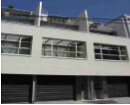
richmond wangaratta street richmond wangaratta street 20
