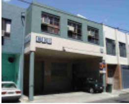
richmond wangaratta street richmond wangaratta street 21
