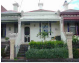
carlton north station street carlton north station street 550
