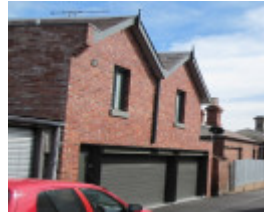
Rear of 76 Wilson Street.jpg
