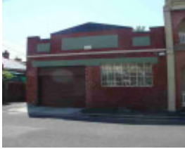
carlton north hughes street carlton north hughes street 26
