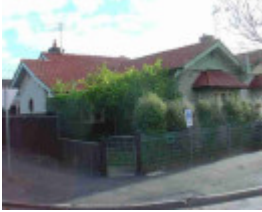
clifton hill fenwick street clifton hill fenwick street 73
