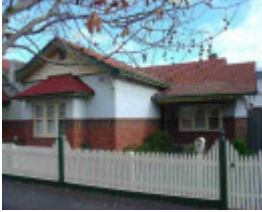
clifton hill fenwick street clifton hill fenwick street 75
