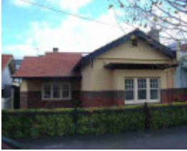
clifton hill fenwick street clifton hill fenwick street 77
