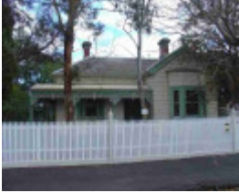
clifton hill fenwick street clifton hill fenwick street 83
