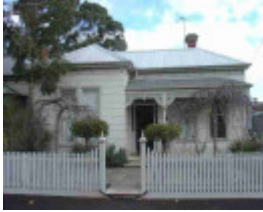
clifton hill fenwick street clifton hill fenwick street 91
