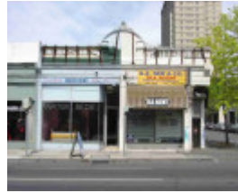
Collingwood Johnston Street 203-205.JPG
