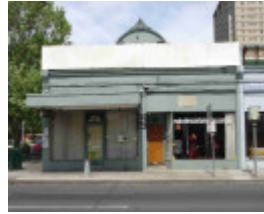
Collingwood Johnston Street 207-209.JPG
