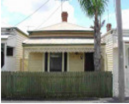
burnley kimber street burnley kimber street 7
