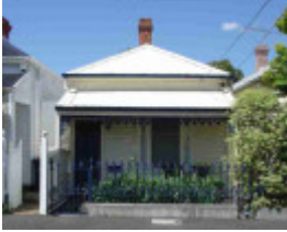
burnley kimber street burnley kimber street 10
