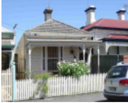
richmond miller street richmond miller street 18
