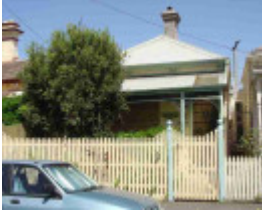
richmond miller street richmond miller street 20
