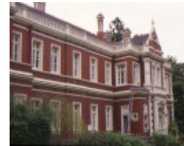
1888 building university of Melbourne parkville side elevation
