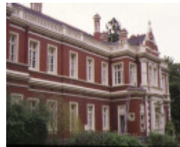
1888 building university of melbourne parkville side elevation
