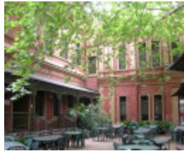
1888 BUILDING, PART OF FORMER MELBOURNE TEACHERS COLLEGE SOHE 2008
