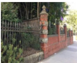
2019 Grattan Street fence.jpg
