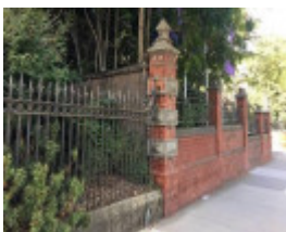
2019 Grattan Street fence.jpg
