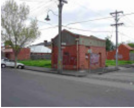
collingwood hotham street collingwood hotham street 64a
