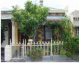
carlton north station street carlton north station street 658
