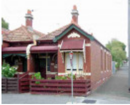
princes hill pigdon street princes hill pigdon street 263
