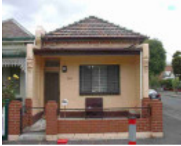
carlton north station street carlton north station street 587
