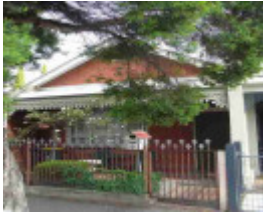
carlton north richardson street carlton north richardson street 11
