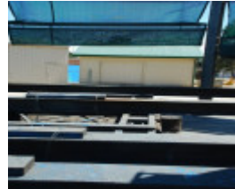
SLIP AND WINCH SHED SOHE 2008
