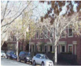
Cable Tram Engine House
