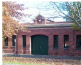
Cable Tram Engine House
