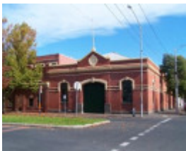
Cable Tram Engine House
