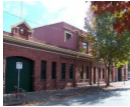
Cable Tram Engine House
