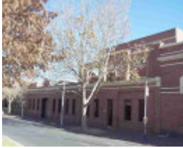
Cable Tram Engine House - 1023 Rathdowne
