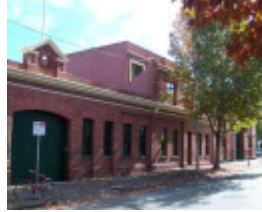
Cable Tram Engine House
