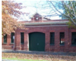
Cable Tram Engine House
