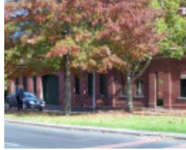
Cable Tram Engine House
