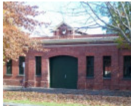
Cable Tram Engine House
