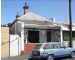
richmond wangaratta street richmond wangaratta street 16
