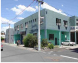
richmond wangaratta street richmond wangaratta street 17-19
