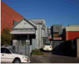
clifton hill roseneath street clifton hill roseneath street 118 unit 5
