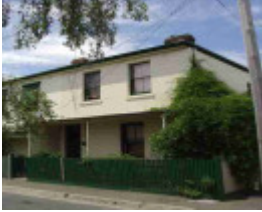
richmond tyson street richmond tyson street 9
